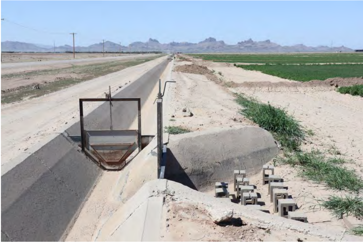
West view of south concrete lined ditch
