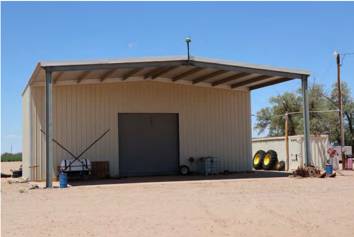
Shop building 2500 s.f. metal over concrete, 50% enclosed
