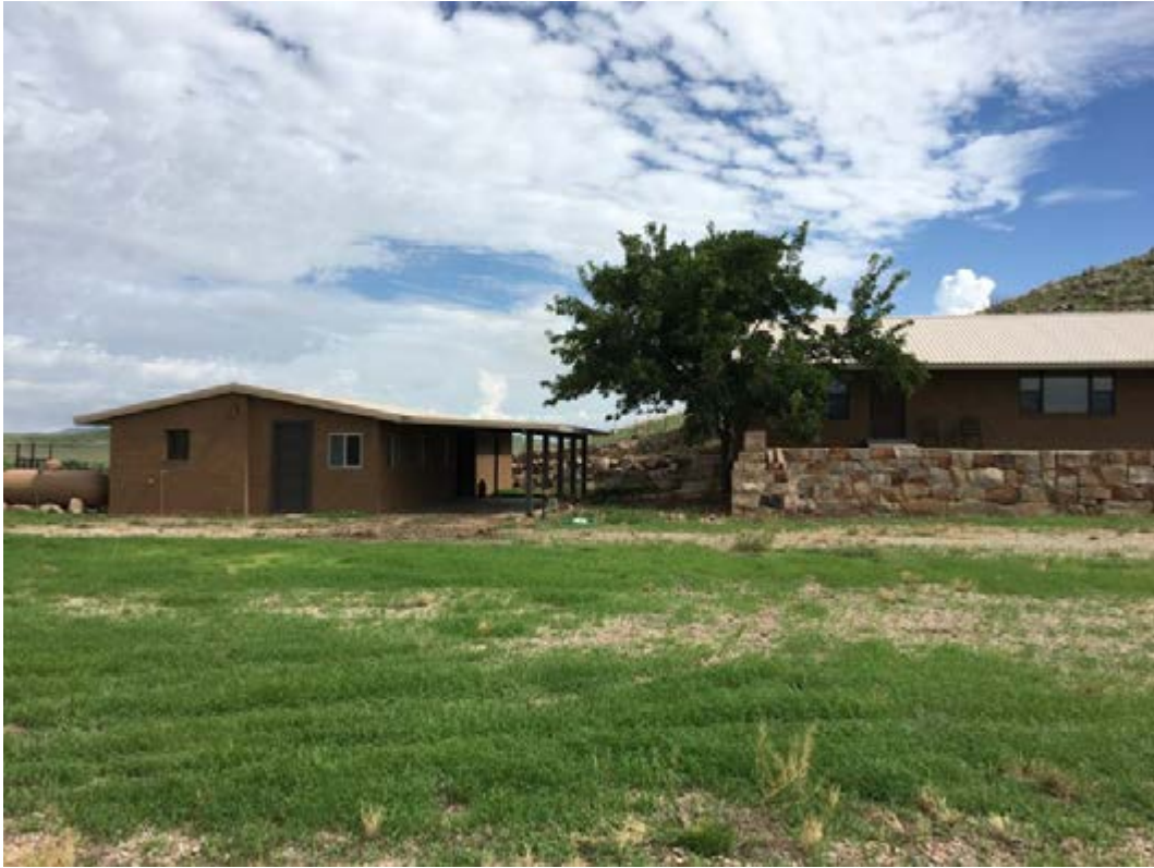
Residence and bunkhouse
