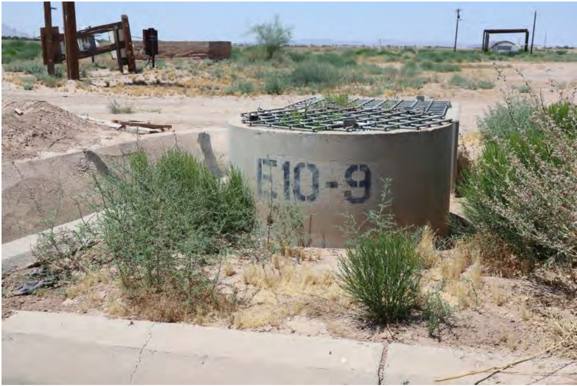
MSIDD water delivery turn-out
