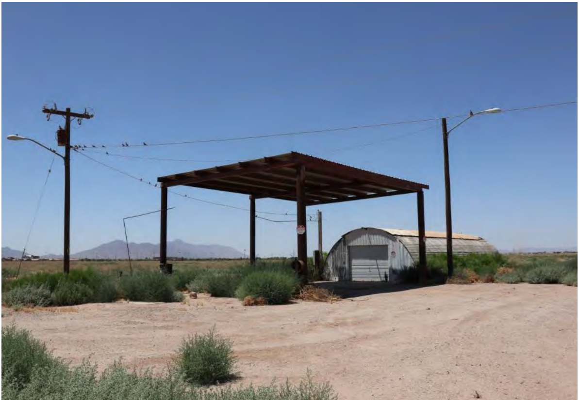
Shop building improvements
