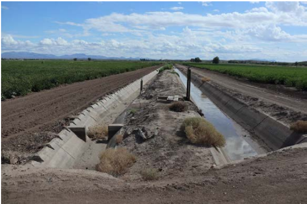
Montezuma Canal turnout and typical notched farm ditch
