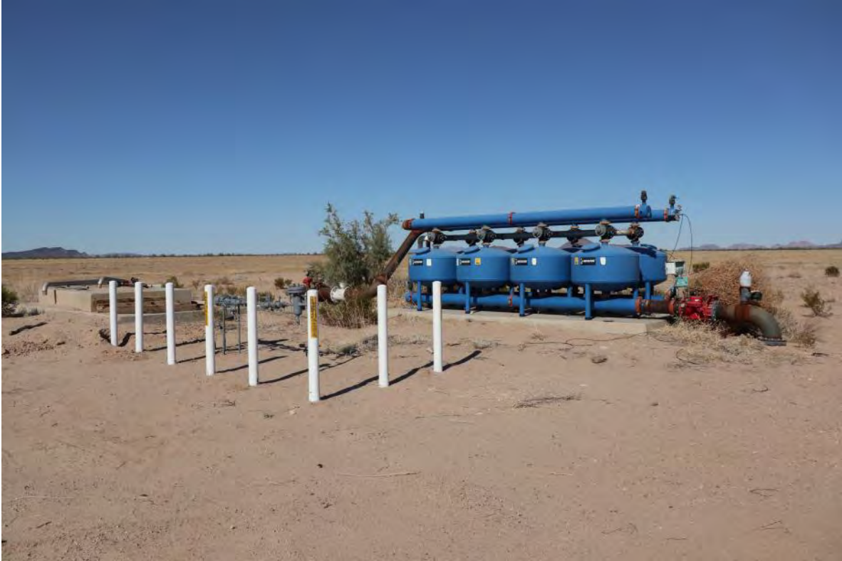
Sand media filtration at Bassett well site 6
