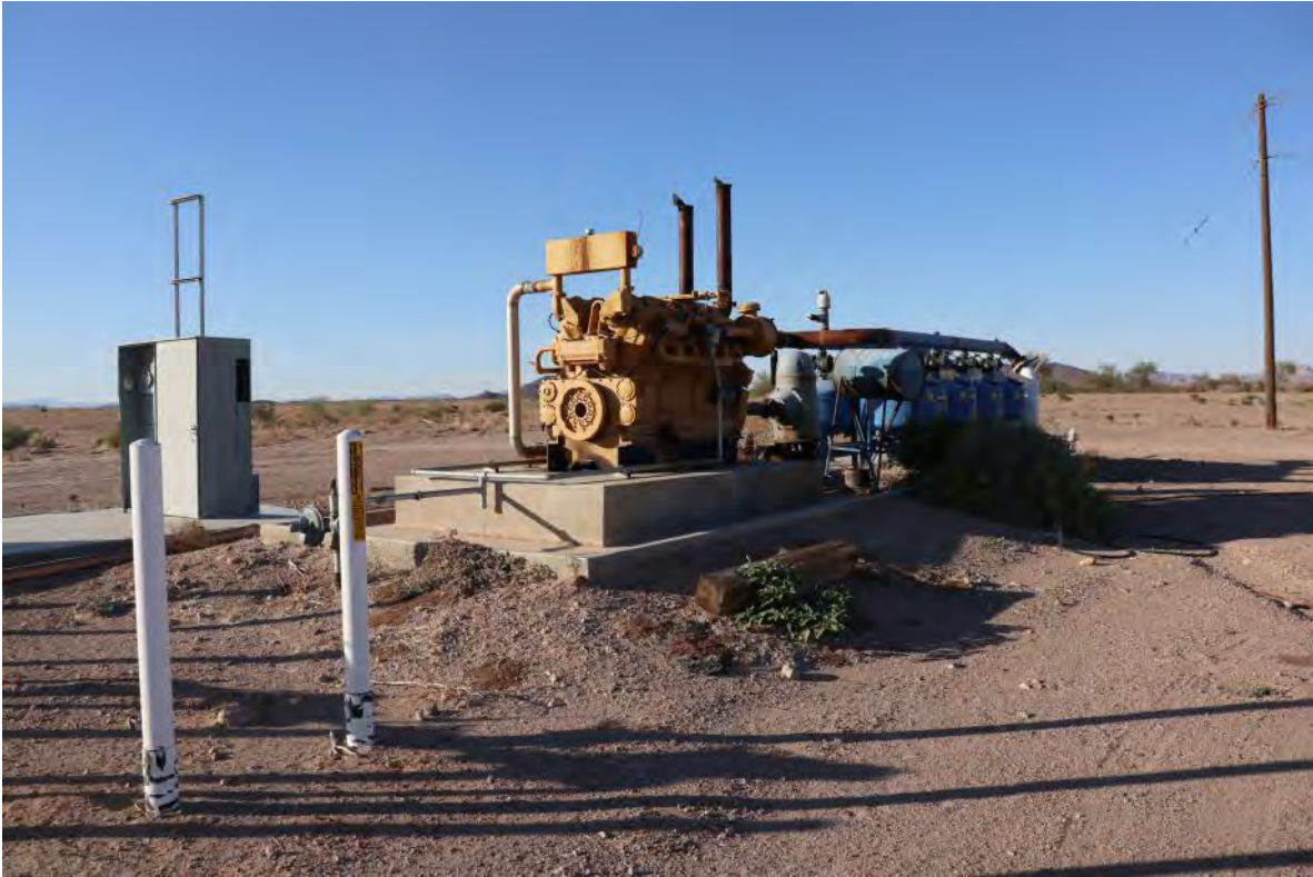
Natural gas engine Mille Verde well site 5
