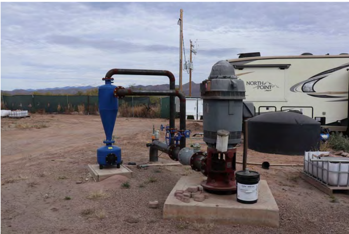
Well 1,005' deep, 12-3/4" casing, 150 hp, 600-650 gpm
