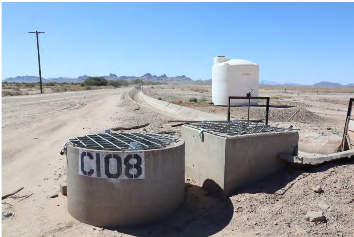
Irrigation district turn-out, CAIDD C108
