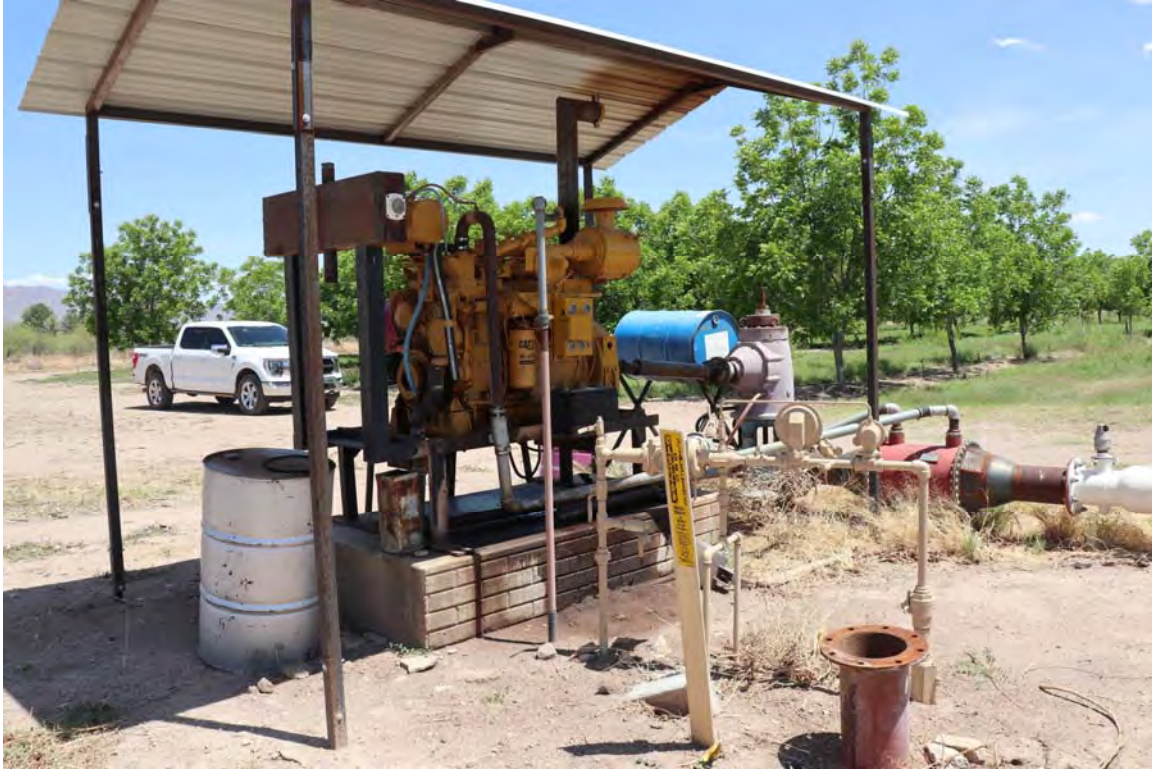
North well, natural gas driven irrigation pump
