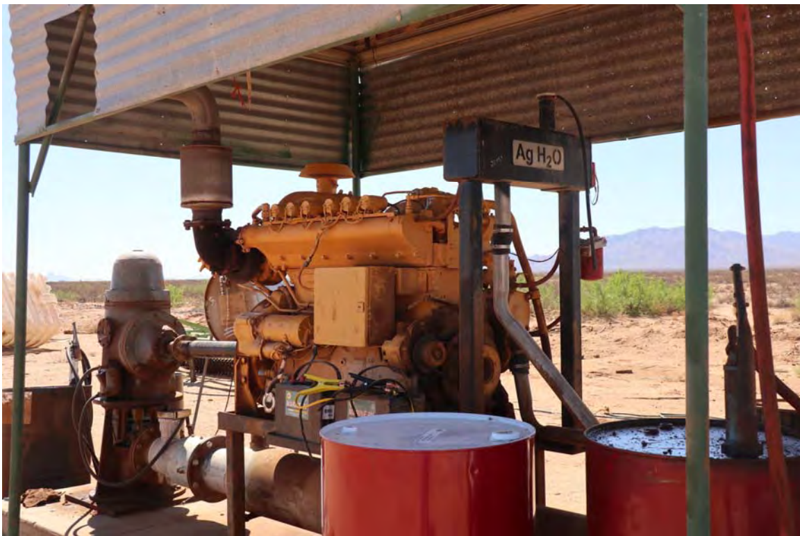
Irrigation well 1,200' deep, 1,100 GPM capacity, CAT 3406 gas engine
